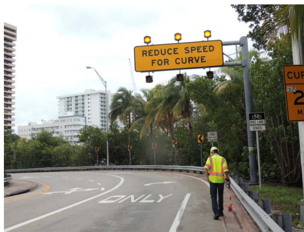
FIGURE 3 – HFST on Tight Curve before a Signalized Intersection.
